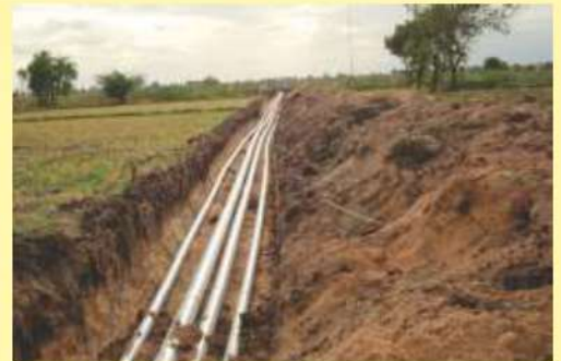
Installation of Supreme pipeline in the field
